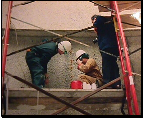
Exposed Aggregate Beam Repair
