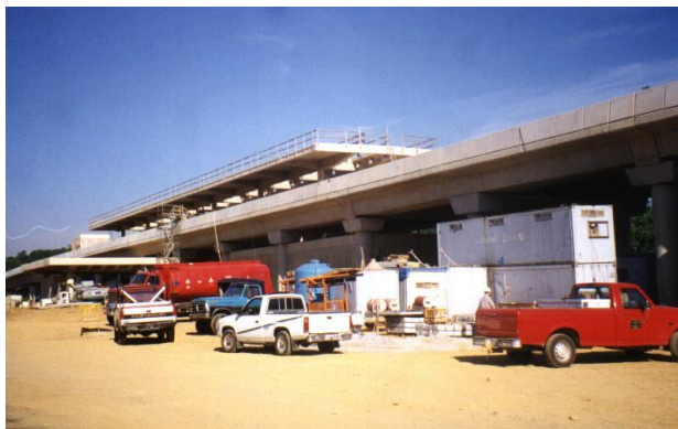
WMATA - Naylor Road Station
