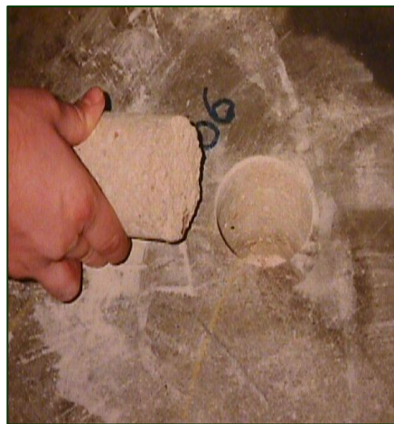
Core examination of rebonded topping slab
